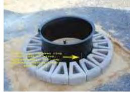
**4 Once correct positioning has been established for the first layer, remove the ring and place to the side.**
