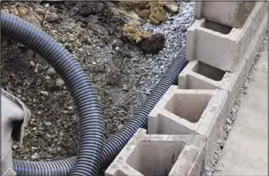
Drainage Pipe Placement
