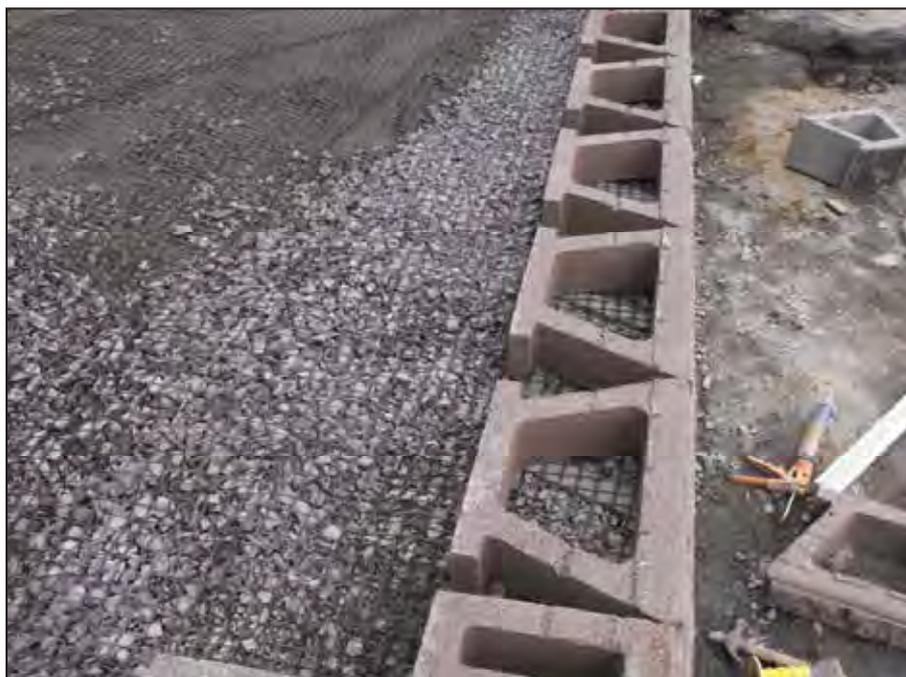
Drainage Aggregate (Inside and behind units)
